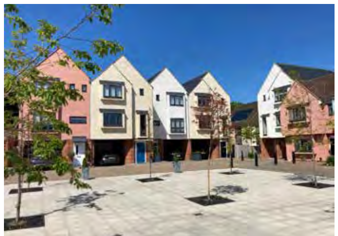
Old Station Close
