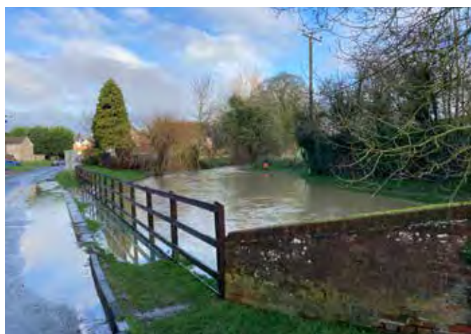
Flooding at the end of Prentice Street
