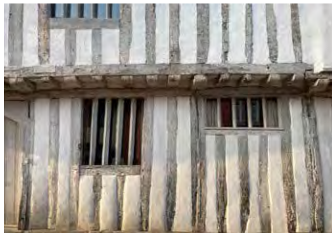
Timber facade of The Priory
