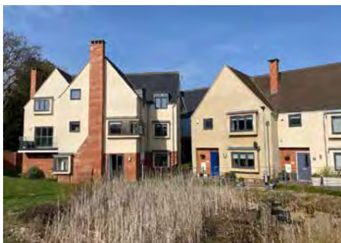
Old Station Close
