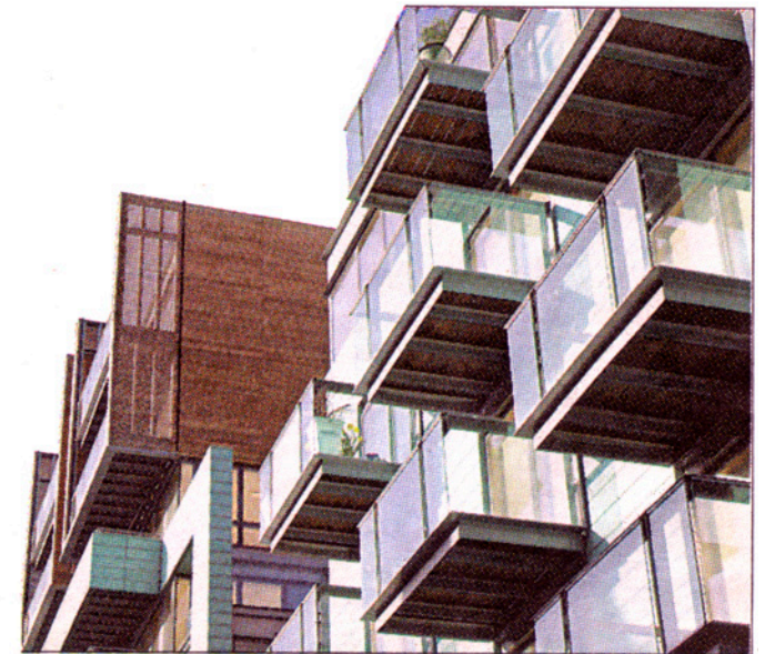
High society: the nine-storey development by Peabody Trust in Nile Street, N1, aims to attract a mix of key workers and young City types with its striking turquoise copper cladding and spacious balconies
